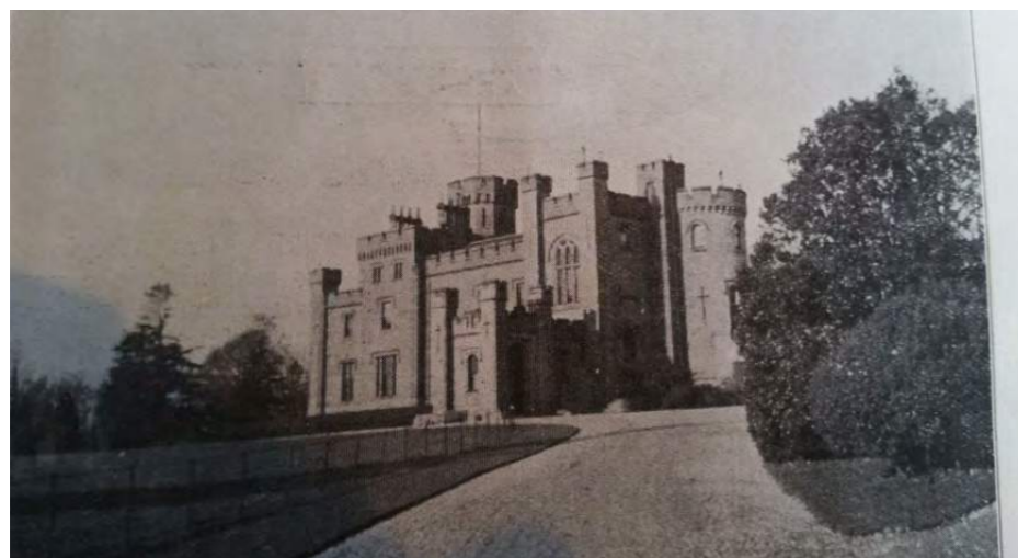
Mansion house in its initial form by David Hamilton
